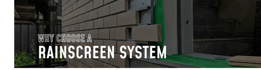
As the world increasingly turns to more sustainably designed builds, Fairview is investing substantially in the development of rainscreen cladding systems for both our natural and metal product ranges. Rainscreen facade is a two-level construction system which provides superior waterproofing, long term durability and thermal efficiency.
